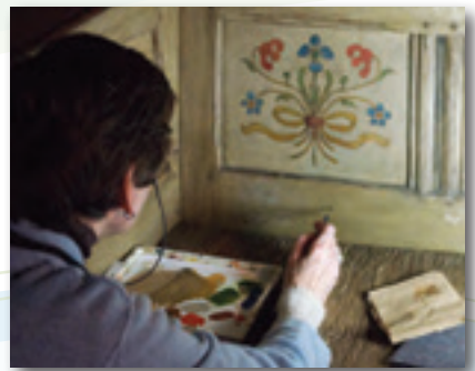
Restoration begins on the West Porch with in-painting and the creation of replicated cushions on the built-in benches.
