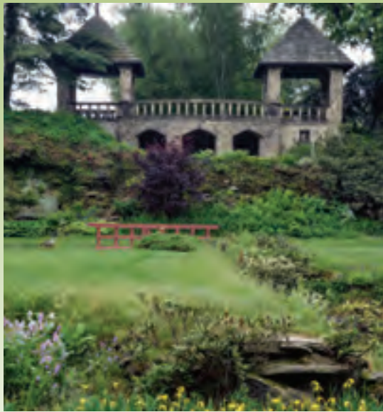
The cliff face is being stabilized to protect the Tea Houses and Hidden Aspect.
